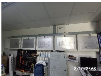
Graphic Annunciator Fire Alarm System
